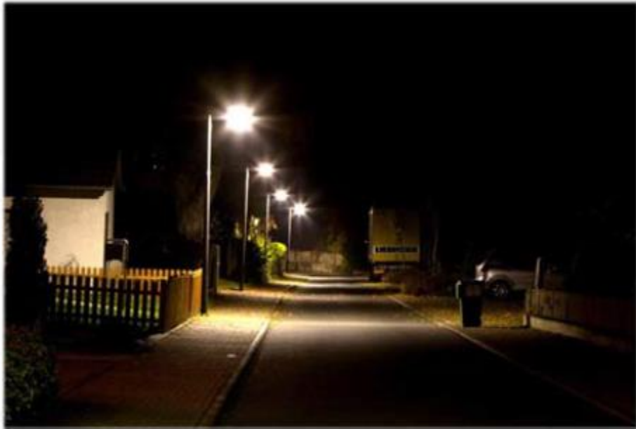
Fig. 4 a: Metal Halide Lighting Used before Replacement
