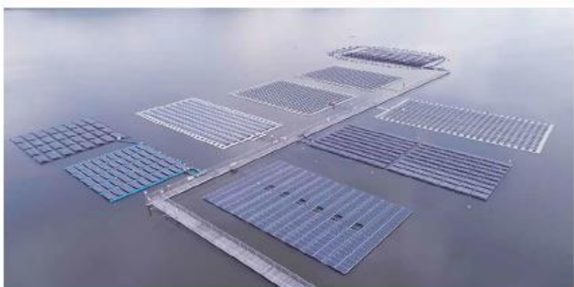
50 MW Tengoh - Singapore
