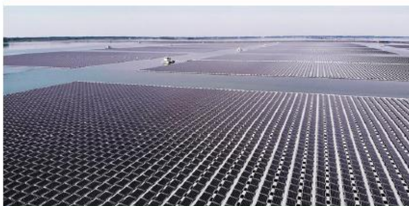
150 MW Guqiao - China
